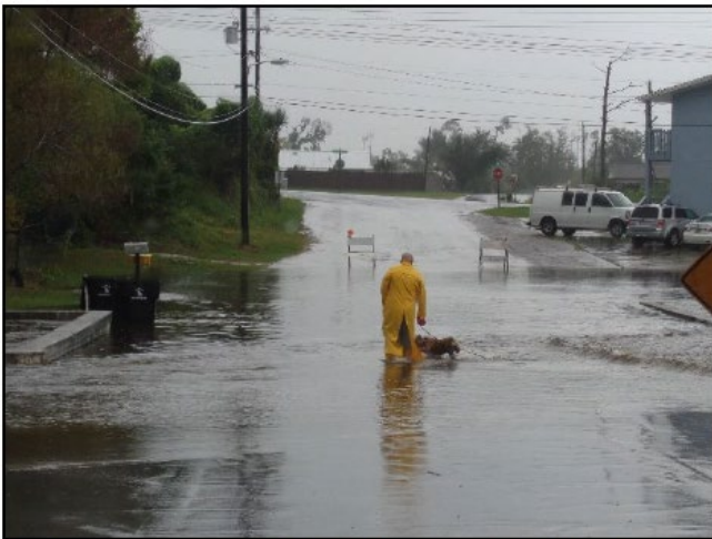
Roadway overtopping at East 5 th St. during September 2020 flood event. Photo courtesy of City of Springfield.
